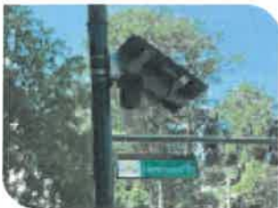
Solar and Existing Pole
